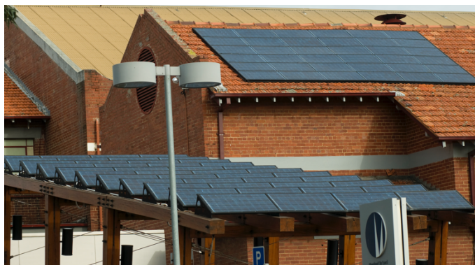
Figure 4. Solar panels in the City of Moreland (photo by Alexi Lynch).
